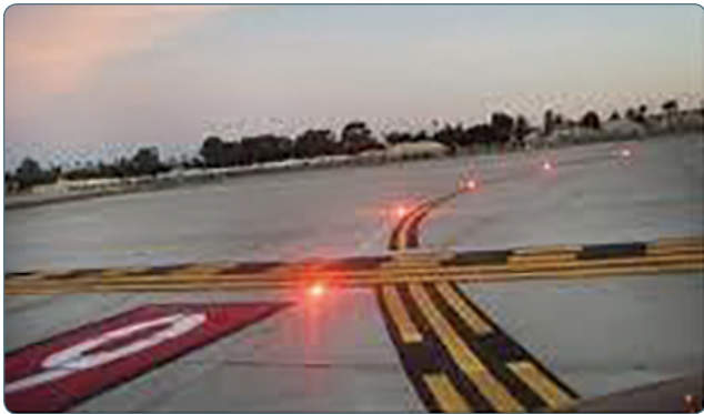
Figure 14-35. Runway Entrance Lights (REL).
